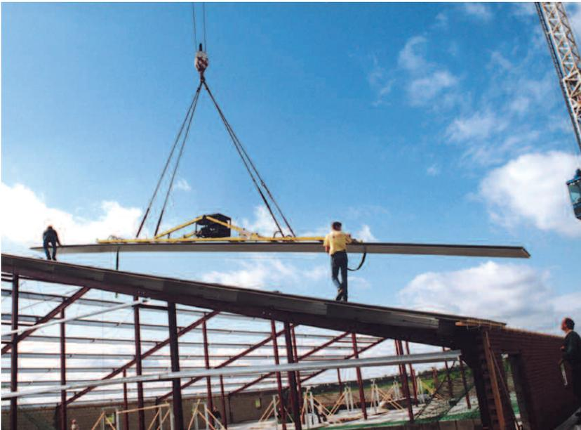
Genugten Agri B.V. also supplies various sandwich panels for roofing and wall cladding. These panels are available in various thicknesses and colours. The colours depend on the coating applied to the panels, i.e.: silicon polyester, 200 µm thick HPS or plastisol coating. The panels are available cut to length for lengths up to 16.50 metres. The roofing panels are placed on the roof with a suction cup. The sandwich panels come in
